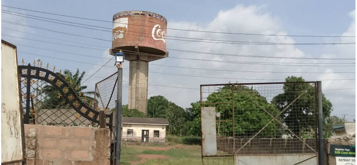
• Ugbowo waterboard abandoned
