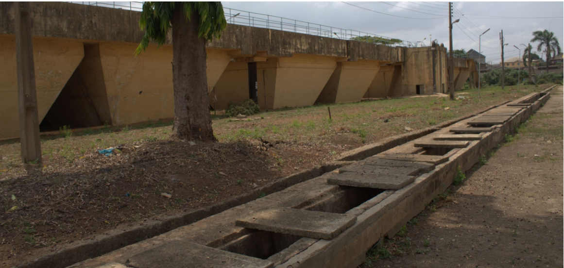
• Empty sedimentation tank in Iju
