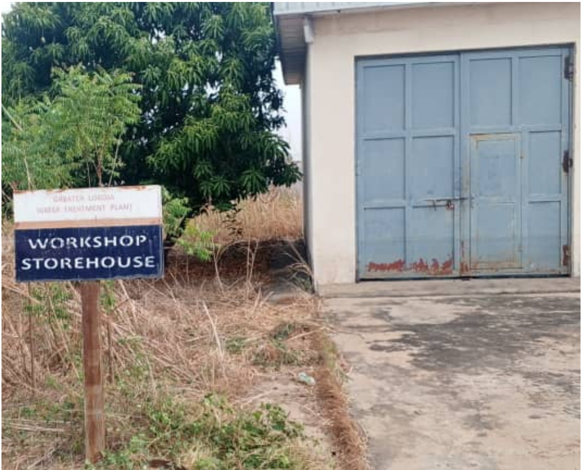
• Workshop storehouse surrounded by weeds
