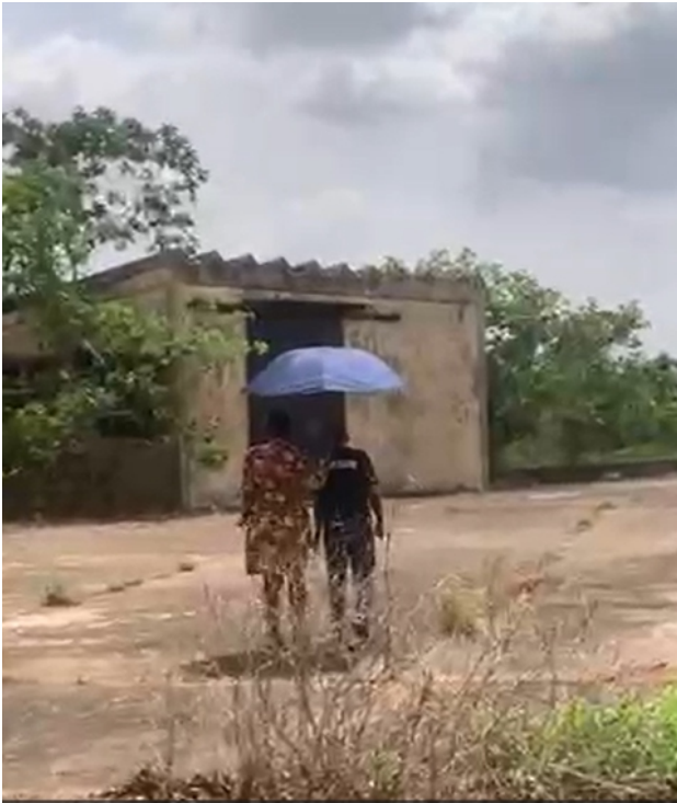
• Abandoned premises at Ikpoba Dam
